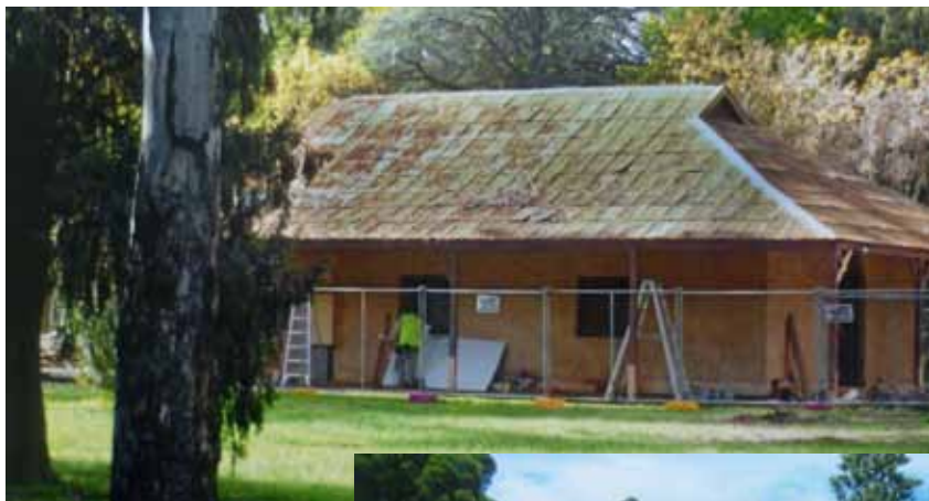
The Tea Rooms being restored...
