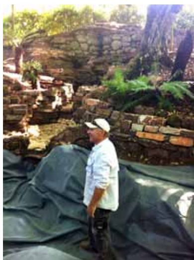
Stonemason at work on the Cascade
